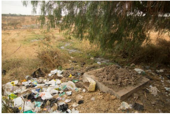
Figure 35 Informal waste dump site and a full overflowing septic tank southwest of gully c, discharging liquid waste into the riverbed.
