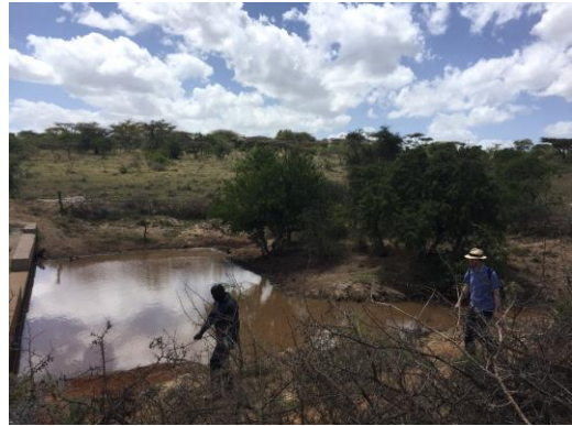
Figure 8 MTTI pilot location shows successful implementation of retention area, serving multiple use water systems.
