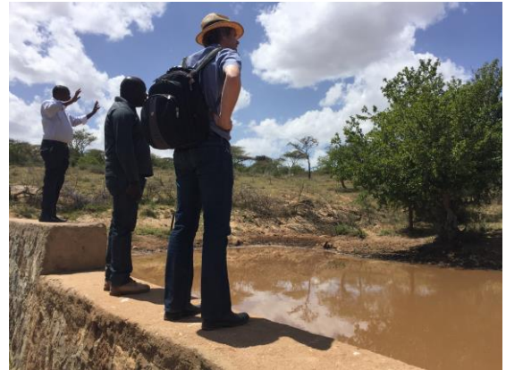
Figure 29 The weir at MTTI storing water
