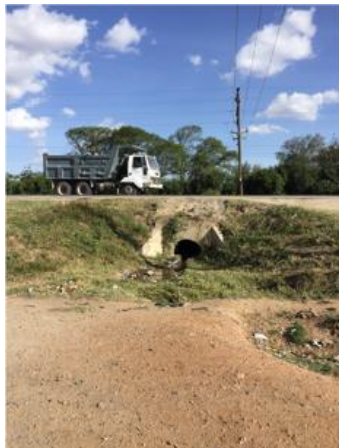
Figure 17 Great north road with the culvert, crossing the road
