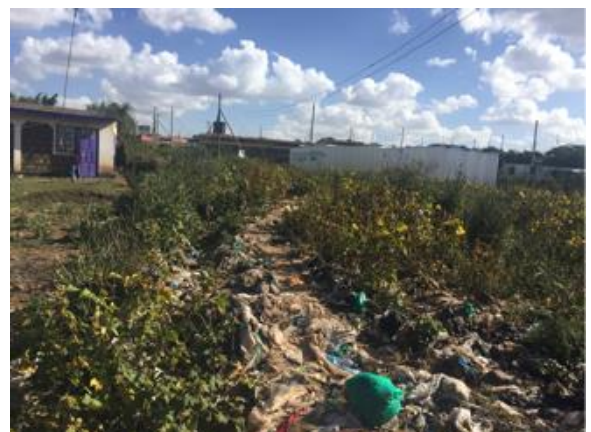
Figure 20 Clogged outer ring gully
