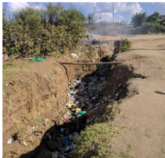
Figure 2 One of the gullies became a dump site
