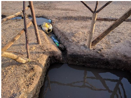
Figure 9: Pilot infiltration pit at a car wash site.
