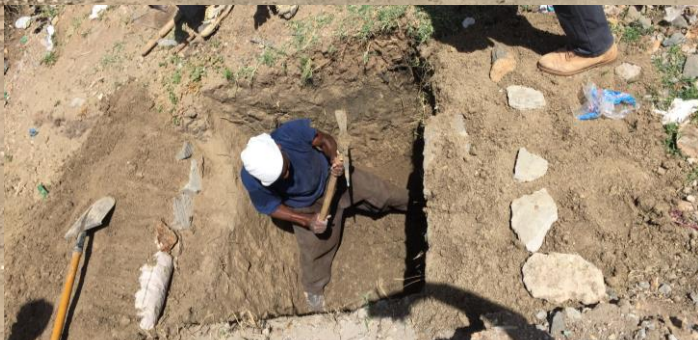
Figure 1 digging an infiltration pit
