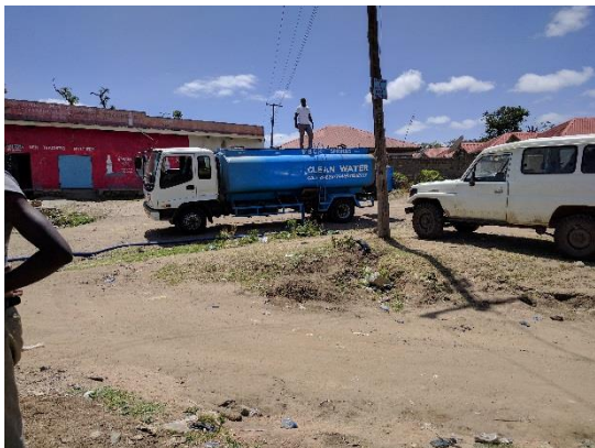
Figure 11: Filling of the SPONGE Infiltration Pit for testing purposes (left) with borehole water from a truck (right).
