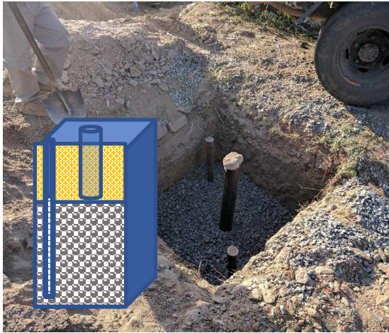
Figure 10: Design and photo of SPONGE Infiltration Pit demo.
